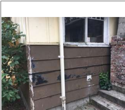
Siding and trim repair
