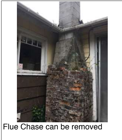
Signs of moisture intrusion
