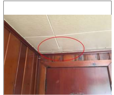
Signs of moisture intrusion above the the door that leads to nowhere.
