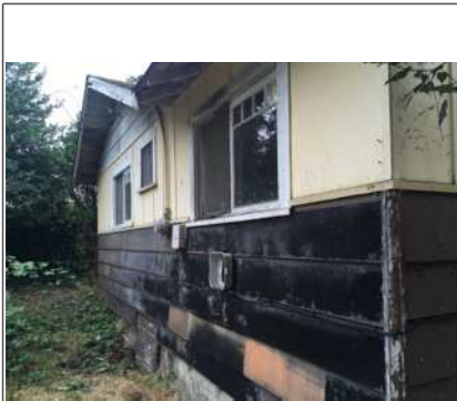
Siding and trim repair
