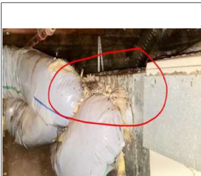
There is a large amount of rodent droppings on top of the furnace.
