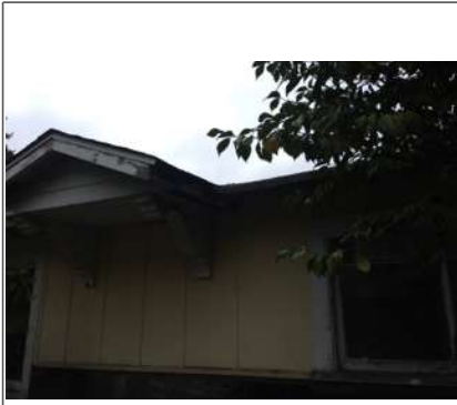
Siding and trim repair
